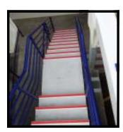
The profiles will also protect the edges of wooden or concrete steps from wear due to knocks and bangs caused by moving equipment.
