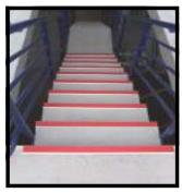
These TredSafe nosings were fitted with Safety Red inserts to offer excellent step edge definition as well as sure footed grip on slippery step edges.
